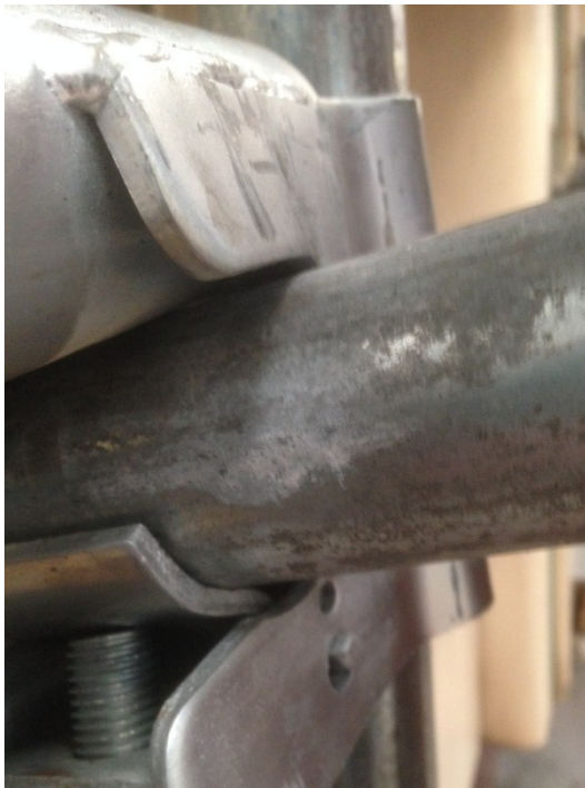
Typical side wall buckling
